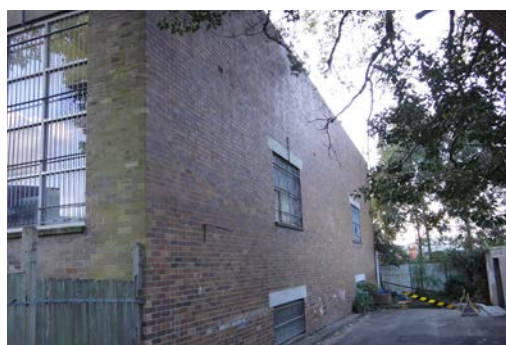
Existing warehouse constructed along boundary in Davies Lane
