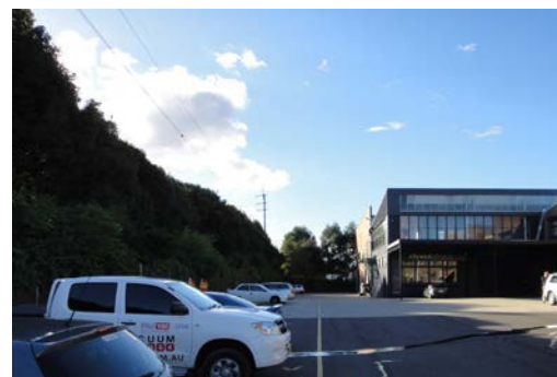
Warehouse and embankment, west side of site
