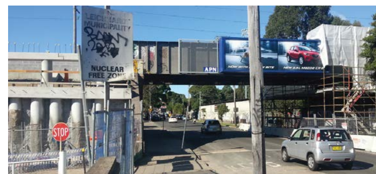
Marion Street Station under construction in June 2003
