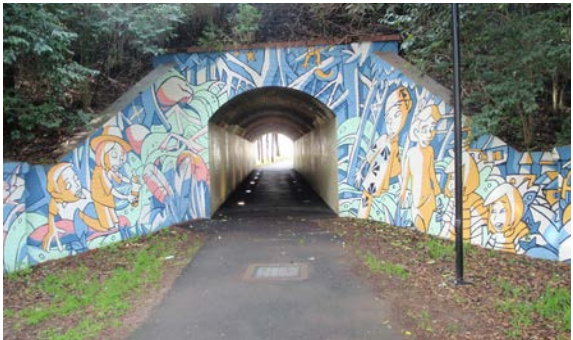
[H] Tunnel under rail embankment
